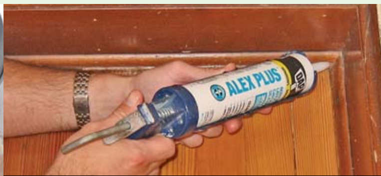
Seal baseboards with caulk
